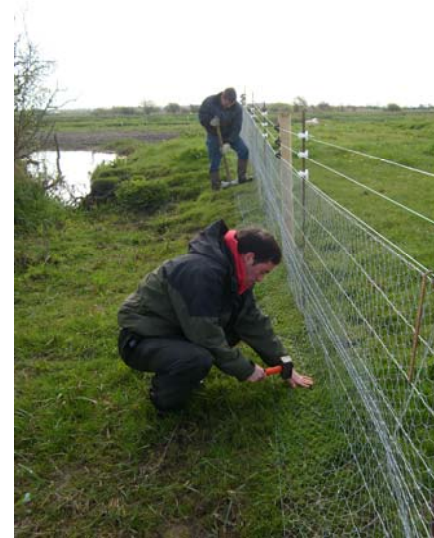
(BirdWatch Ireland volunteers working on a predator proof fence in the midlands)
