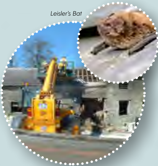
Careful removal of slates will ensure hibernating bats are discovered, and disturbance is minimised
