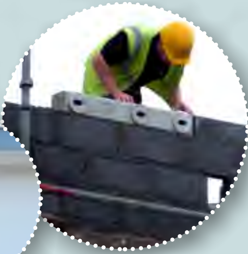
Swift boxes installed at build stage provide suitable nest sites in this new building
