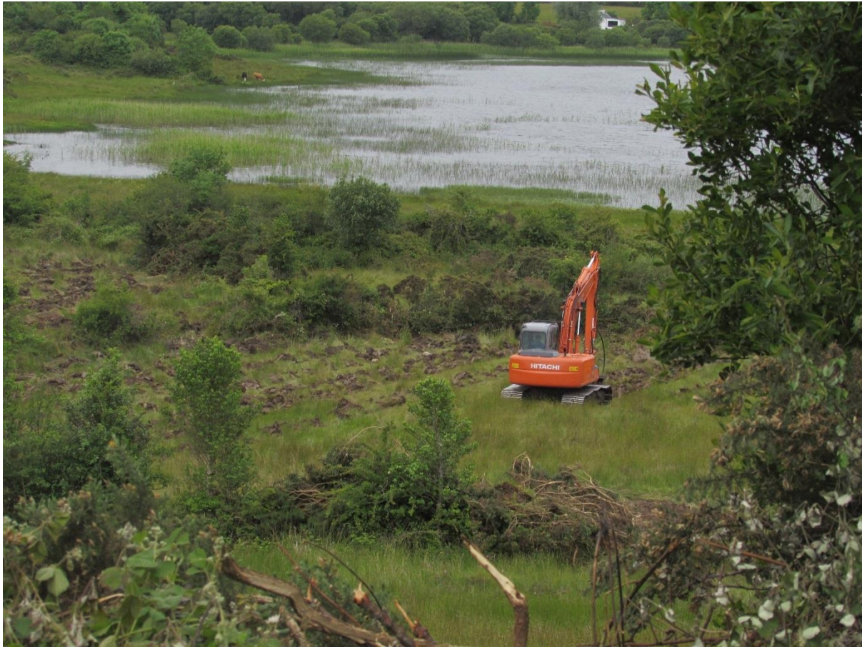
Figure 7. A site in Loughtown Townland, Co. Leitrim which is being prepared for afforestation. The site provided important foraging habitat for Curlew.
