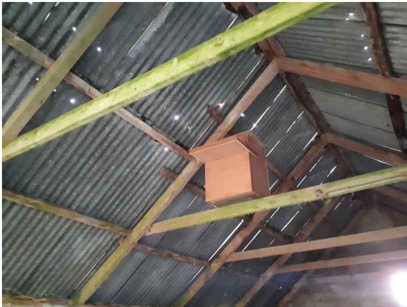
No steel band used with this nest box, it was just screwed onto a platform that was screwed onto the horizontal roof beam, with a few screws securing the lid of the box to the roof beam just above the box (Image: Alan McCarthy)
